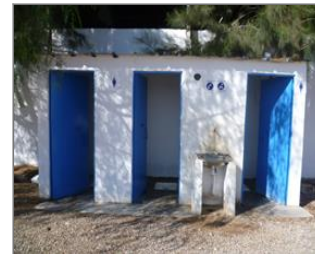
Photo of the sanitary facilities P1040191.JPG
